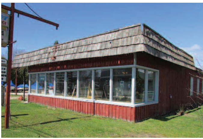
204 WATER STREET • EAST JORDAN
